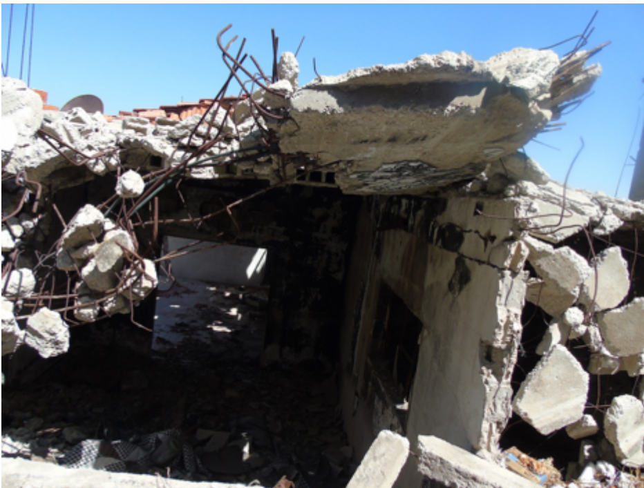
Battle damage at the base of the Krak Des Chevaliers, Syria
